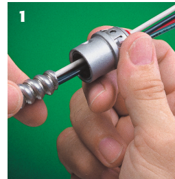
1 Snap fitting onto cable... twist clockwise
