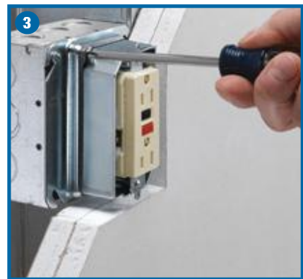
Re-tighten... Adjustment screws.
