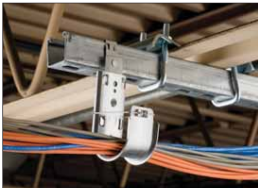
Strut assembly using CATHPESC
