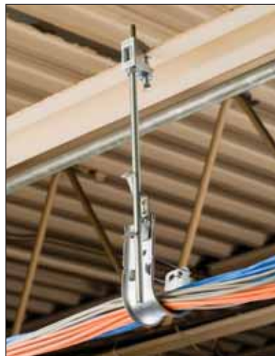
CATHP6Z34 for 3/8" threaded rod and 3/8" - 9/16" flange
