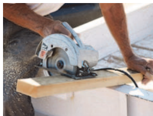
Construction Site Application
