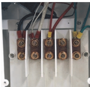
Copper Busbar with Ratings from 250 to 500 A
