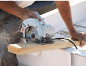
Construction Site Application
