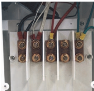
Copper Busbar with Ratings from 250 to 500 A
