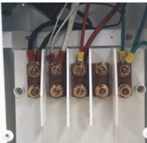
Copper Busbar with Ratings from 250 to 500 A
