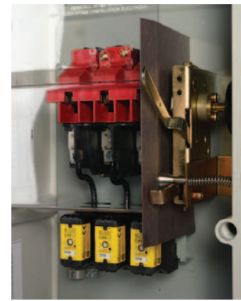
Enhanced Line Shield and Interlock Defeater
