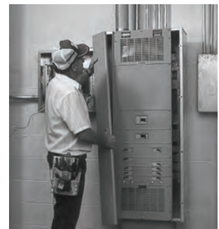
The Three-Piece Trim for Larger Power Distribution Panelboards Provides for Easy Handling and Installation
