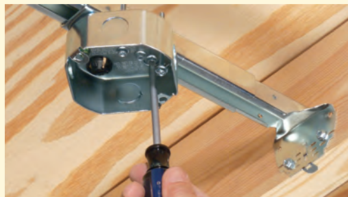
3 Adjust box position from 16" to 24" o.c. between joists.
