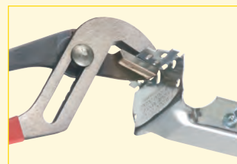
3 Adjust box position from 16" to 24" o.c. between joists.
