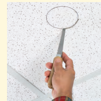
1 Cut a 4-1/16" diameter hole in a 24" ceiling tile.
