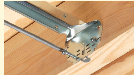
2 Remove screws from both ends of bracket. Use them to attach bracket to joists.
