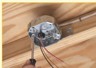
4 Install fan mounting bracket.
