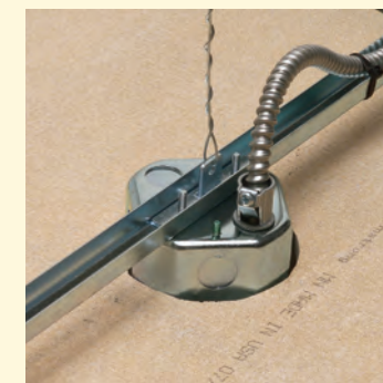
4 Cable pulled through cable connector (not supplied).
