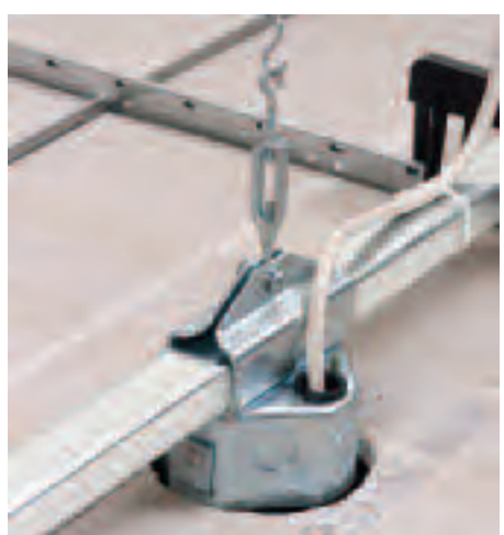
Cable pulled through installed NM cable connector.
