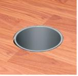
After concrete has cured and finished floor installed,cut the installed concrete box to the finished floor height. If using the low voltage divider, cut the same amount from the bottom of the divider as you removed from the can.
