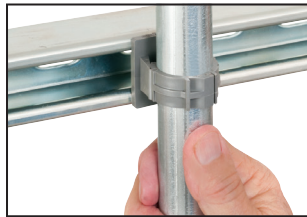
5 Secure installation of conduit to strut.
