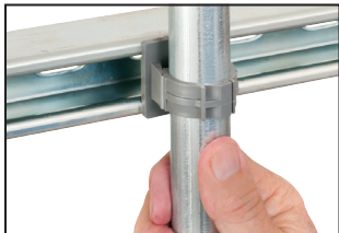
5 Secure installation of conduit to strut.
