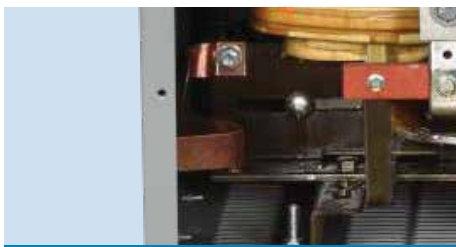
Factory installed main grounding lugs
