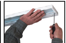
Step 3 Mount fixture to cabinet bottom using captive mounting screws.
