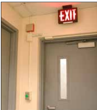
Typical applications for 500 & 700 Series Raceway.
